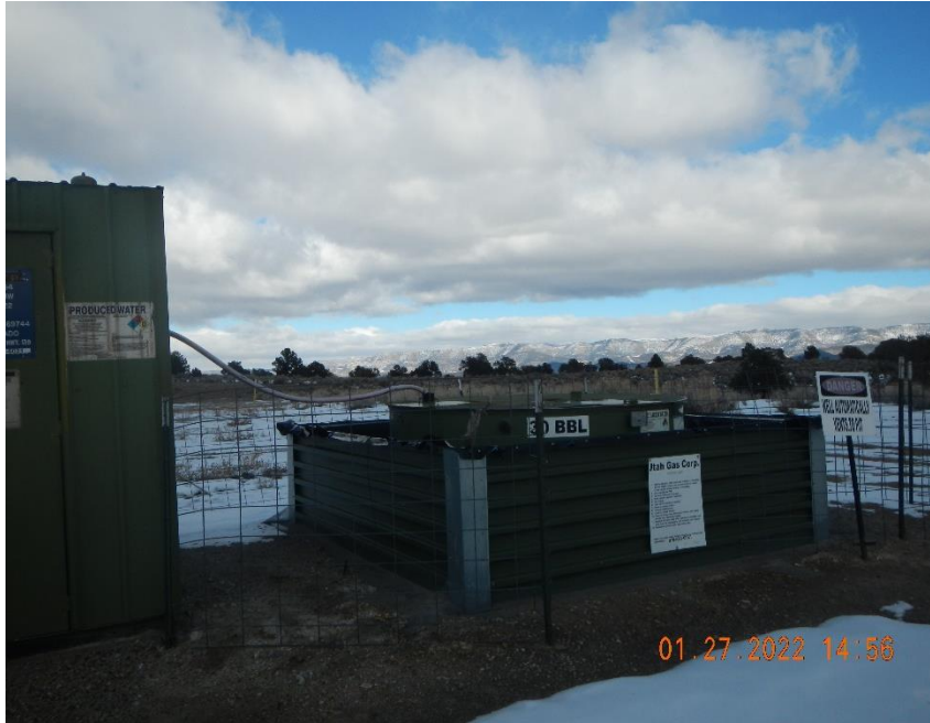
Tank battery sign not at tank battery.
