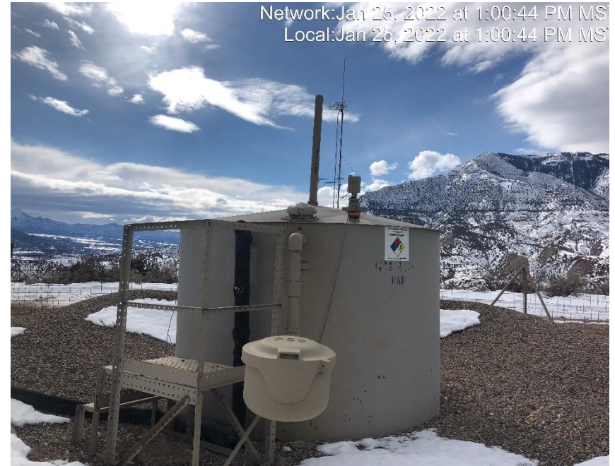
Photo #5781 Vent pipe on tank open ended.
