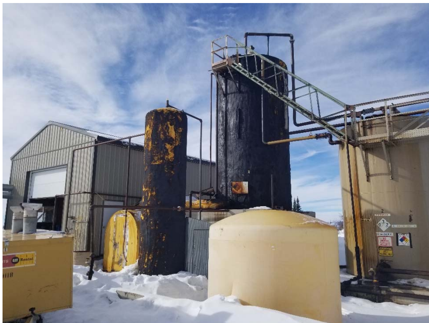
Photo 2. Missing/incomplete tank labels.
