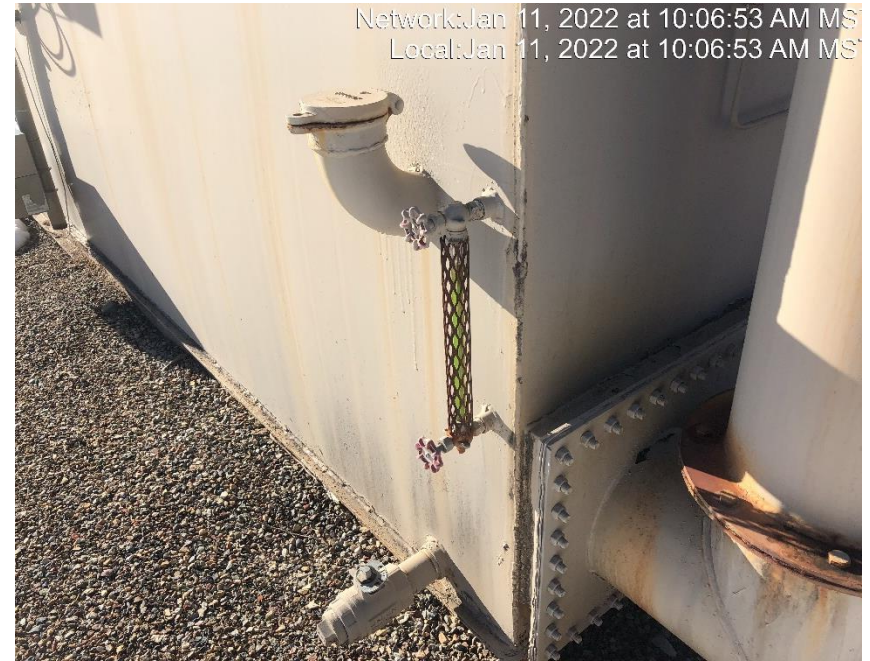
Photo #5638 Sight glass indicates the storage tank is full of an unknown fluid.
