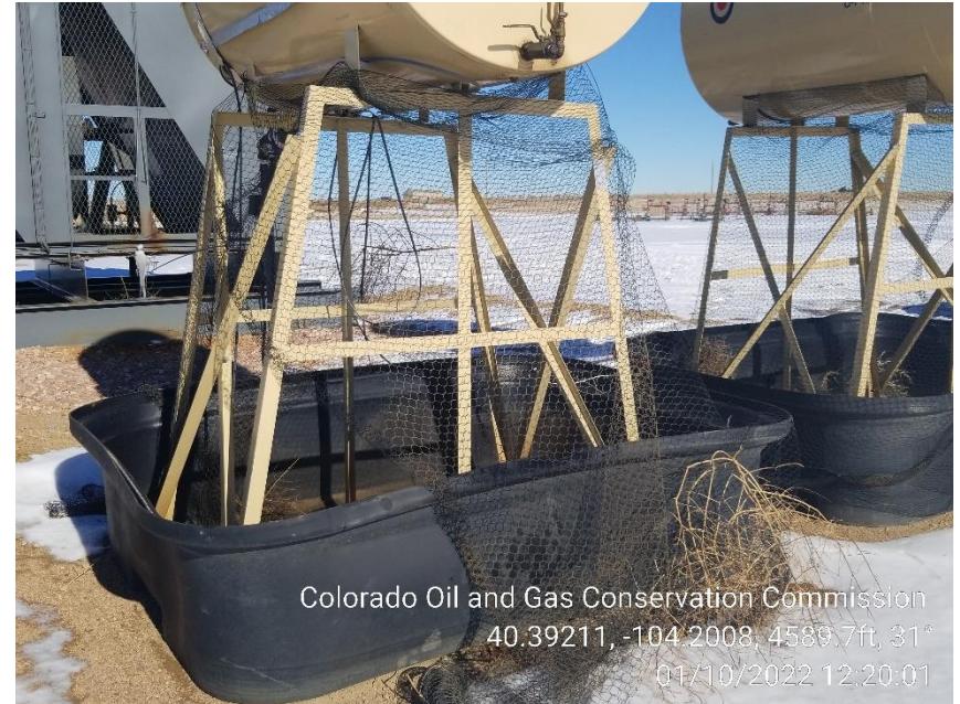
Photo 10 – Day Tank at Compressor Netting in disrepair
