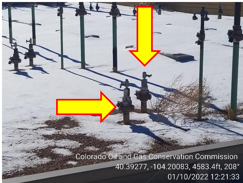
Photo 15 – Unmarked Risers North of Separators
