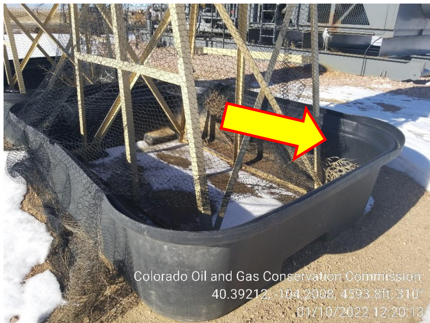
Photo 11 – Day Tank at Compressor Netting in disrepair
