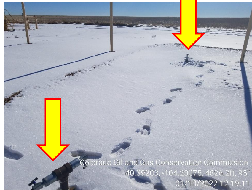
Photo 8 – Unmarked Riser South of Compressor
