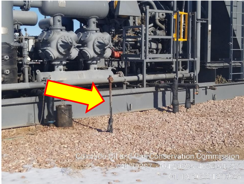
Photo 9 – Unmarked Riser 1" at Compressor
