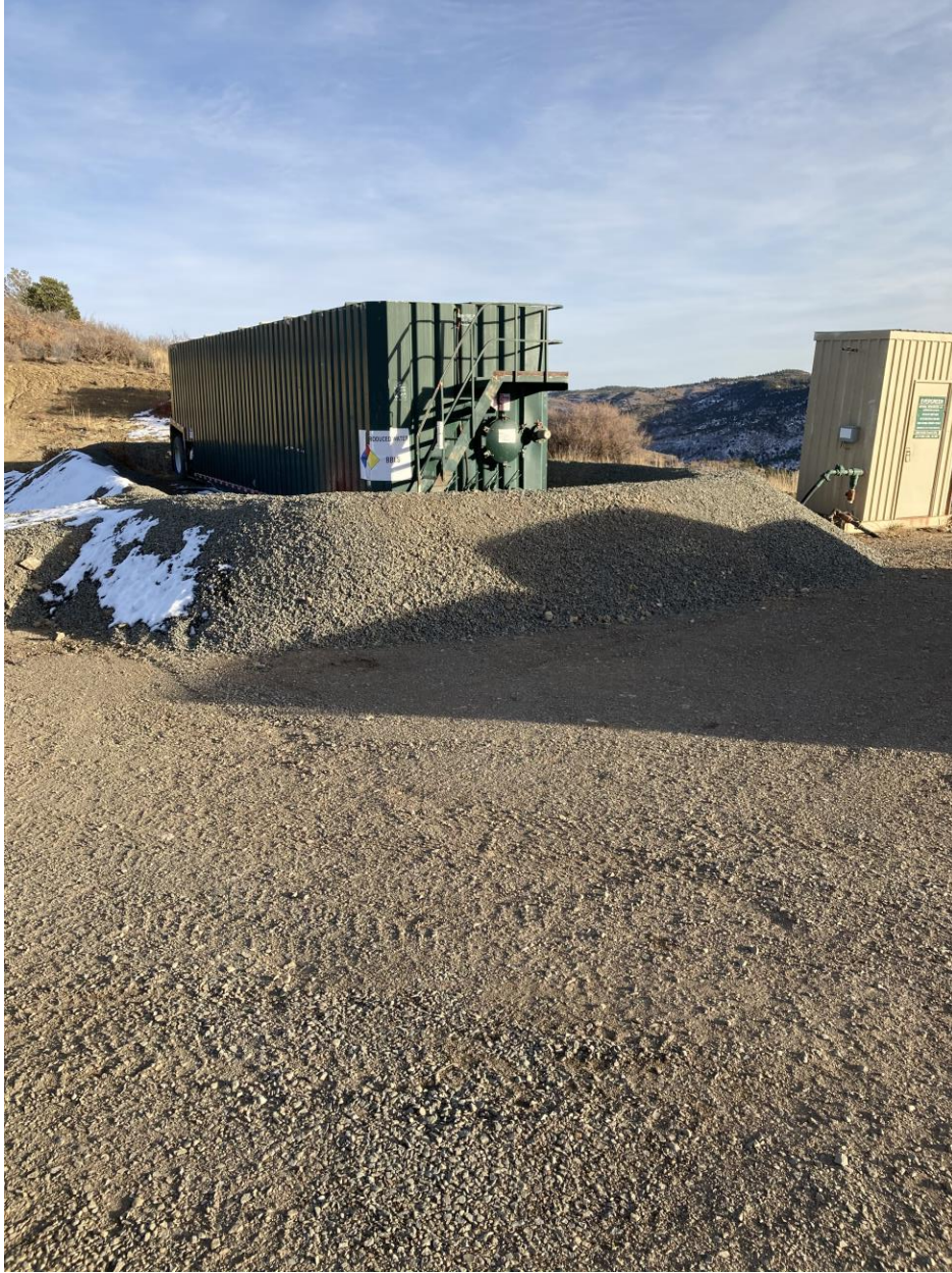
Repaired berm wall in front of tank
