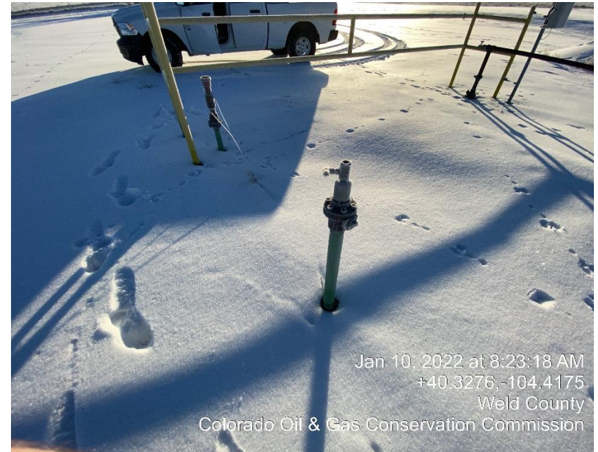
Photo #7 Unmarked Riser
