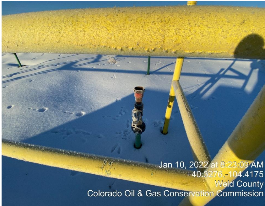
Photo #6 Unmarked Riser
