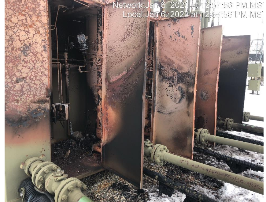
Photo #5609 Separator after fire.
