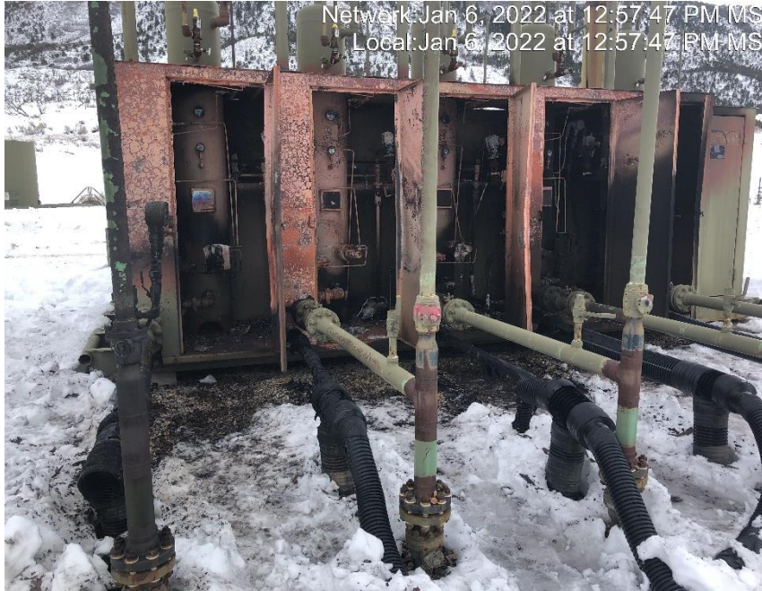
Photo #5608 Separator after fire.
