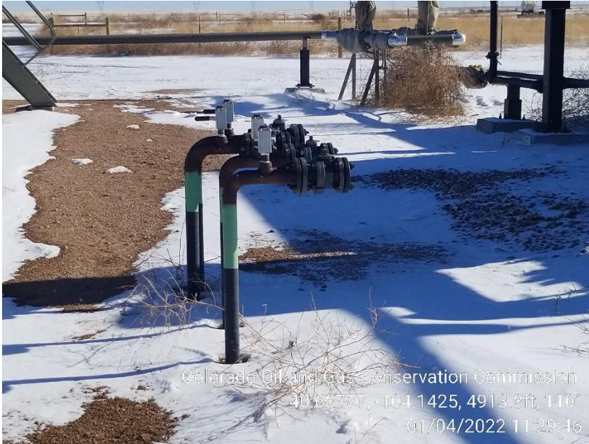
Photo 9 – Unmarked Risers between Separators and Compressor
