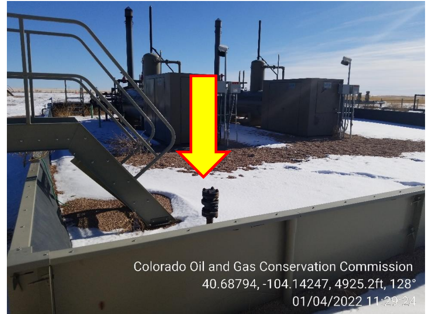
Photo 8 – Unmarked Riser at Separators
