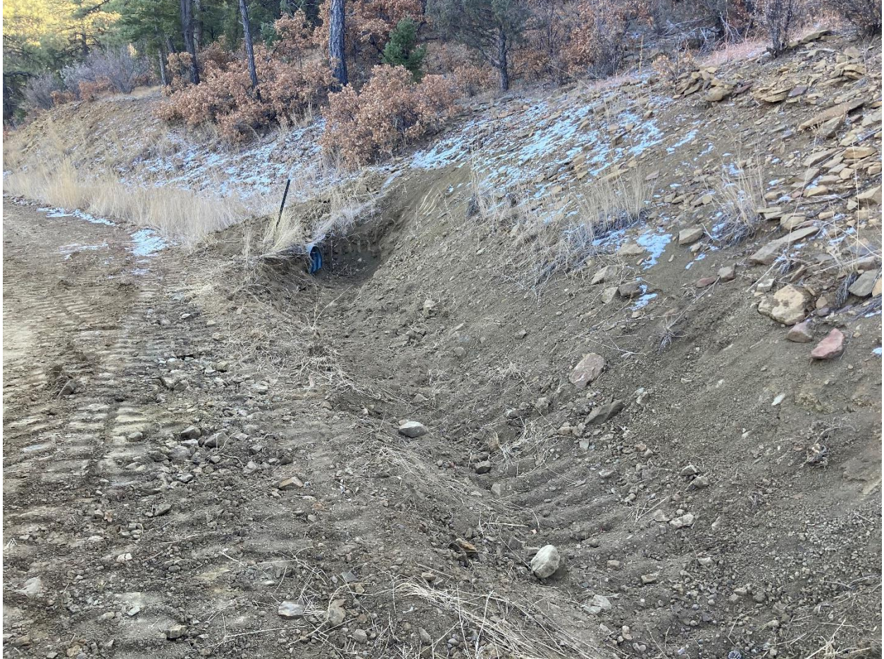
Repaired erosion required BMP's per Rule 1002.f.(2)C
