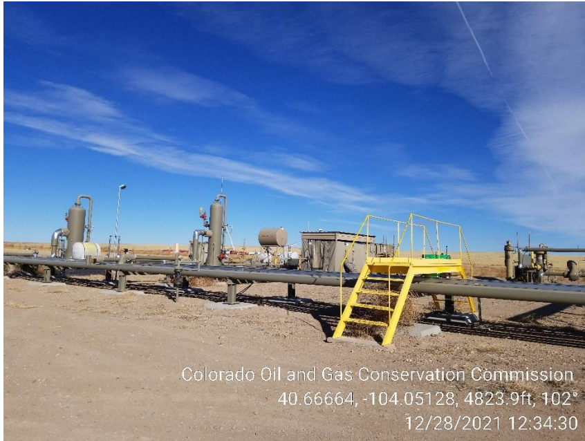
Photo 3 – Compressor and VRU
