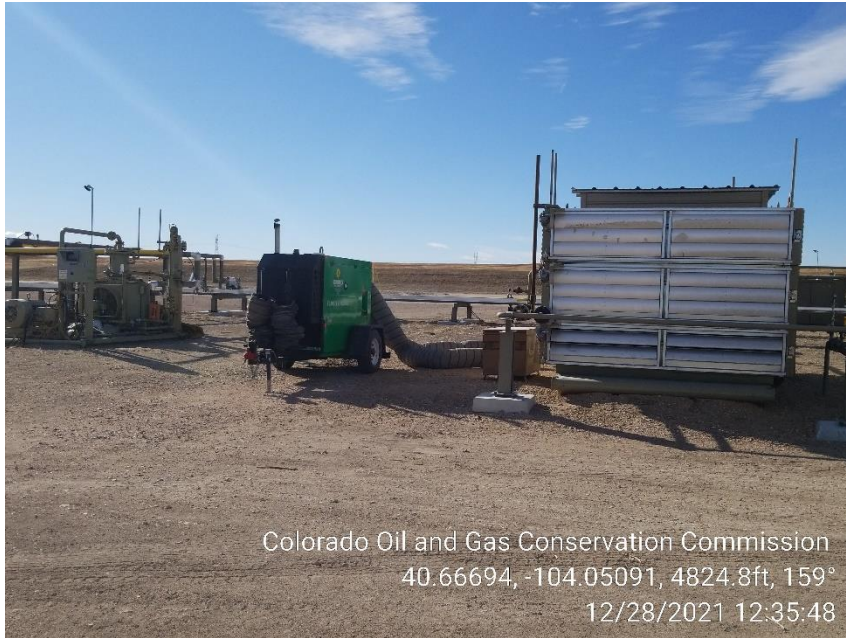
Photo 9 – VRU and Compressor
