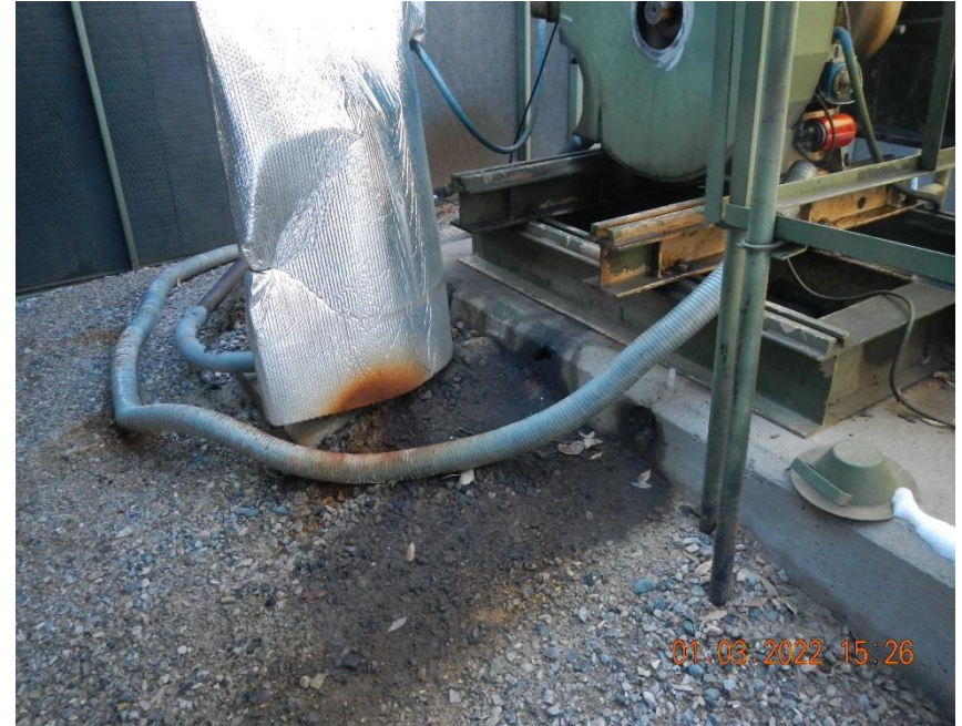
Concrete pad and gravel are wet and stained.
