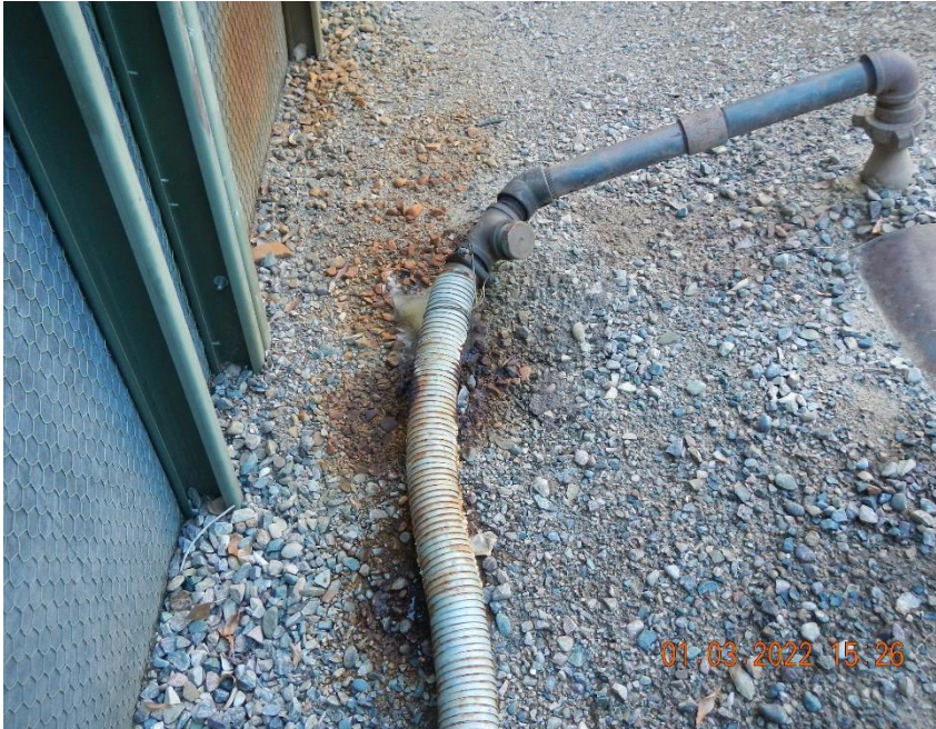
Gravel is stained near exhaust piping.
