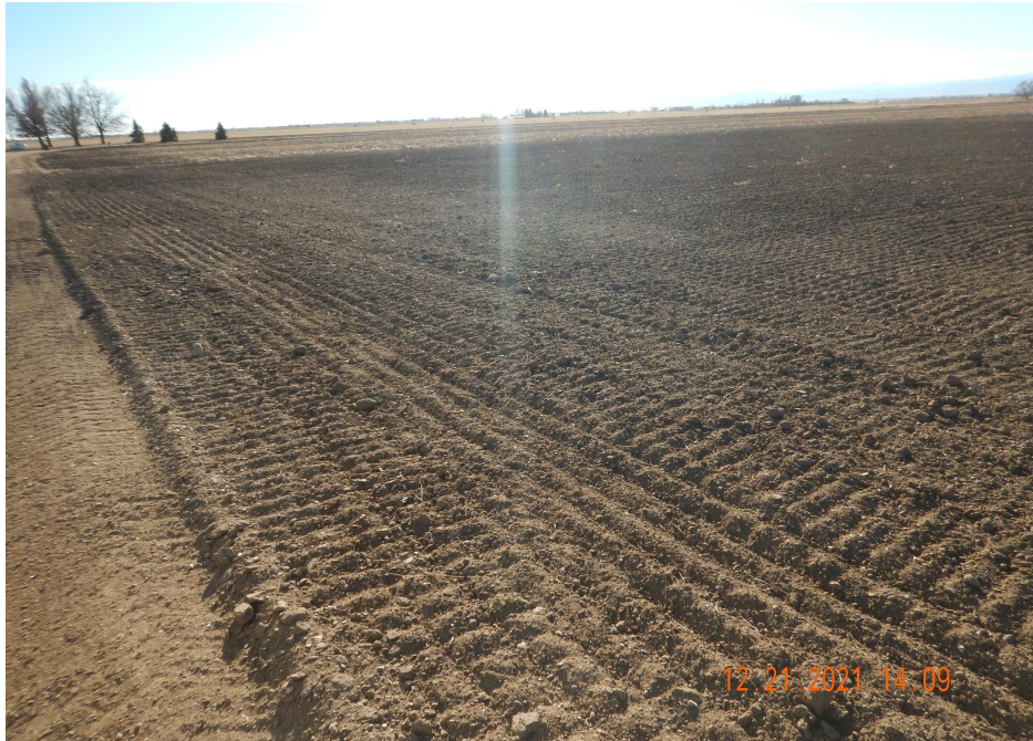
Photo 5. Photo taken from the well location, facing Southwest. Photo illustrates Operator has performed final reclamation activities to remove road base, import topsoil and contour. Staff did not inspect for decompaction.
