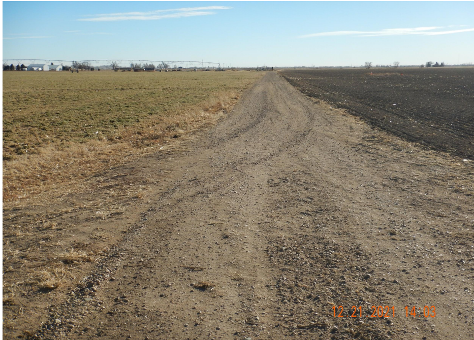
Photo 1. Photo taken from the northwestern well location access road, facing South. Photo illustrates Operator has regraded the access road. There were no observed ruts.
