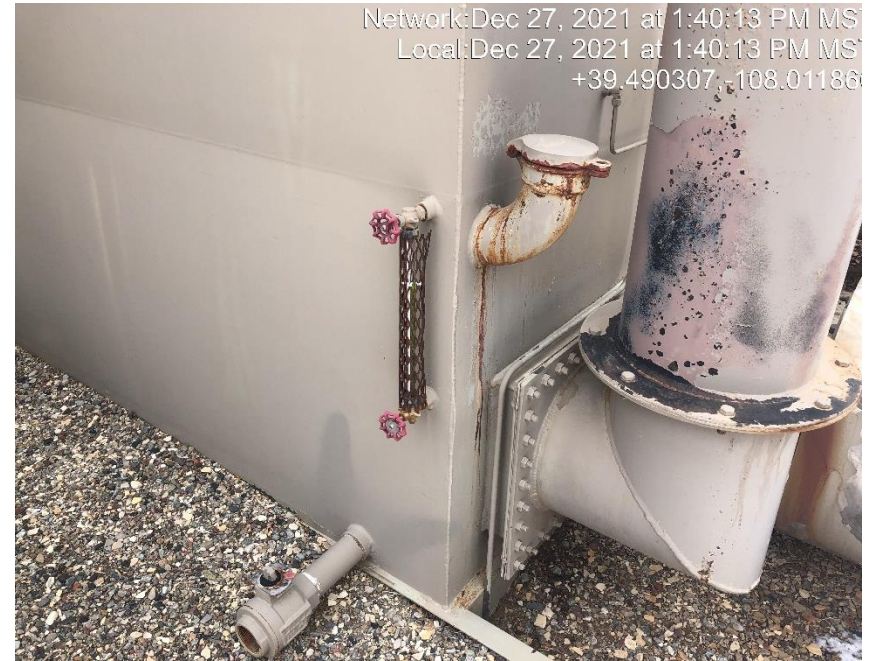
Photo #5521 Sight glass indicates the storage tank is full of an unknown fluid.
