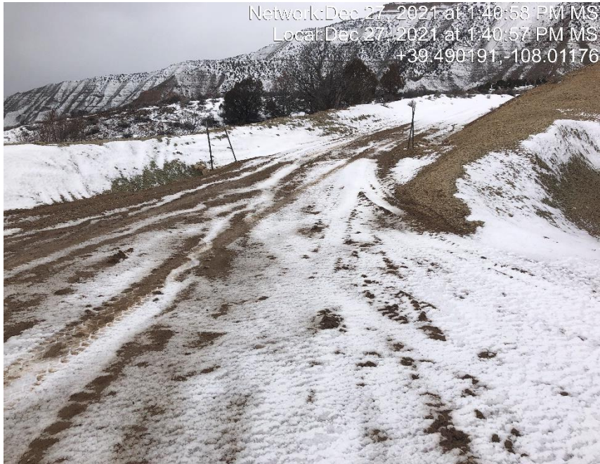
Photo #5524 Insufficient tracking BMP at entrance to location.
