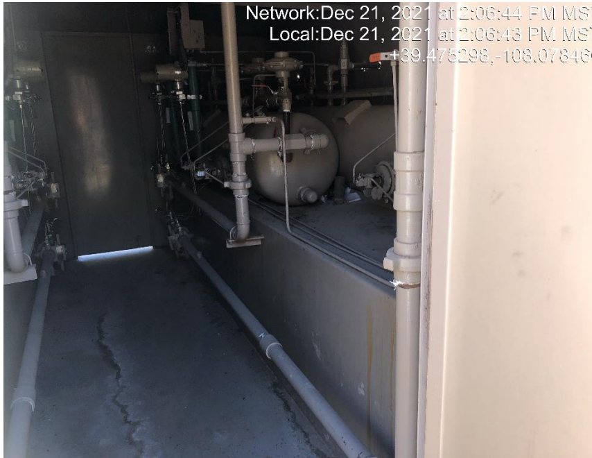
Photo #5484 Storage tank located under horizontal separator.
