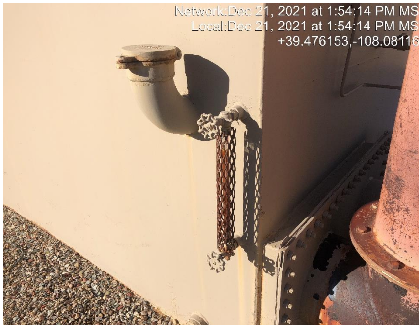
Photo #5475 Sight glass indicates the storage tank is full of an unknown fluid.
