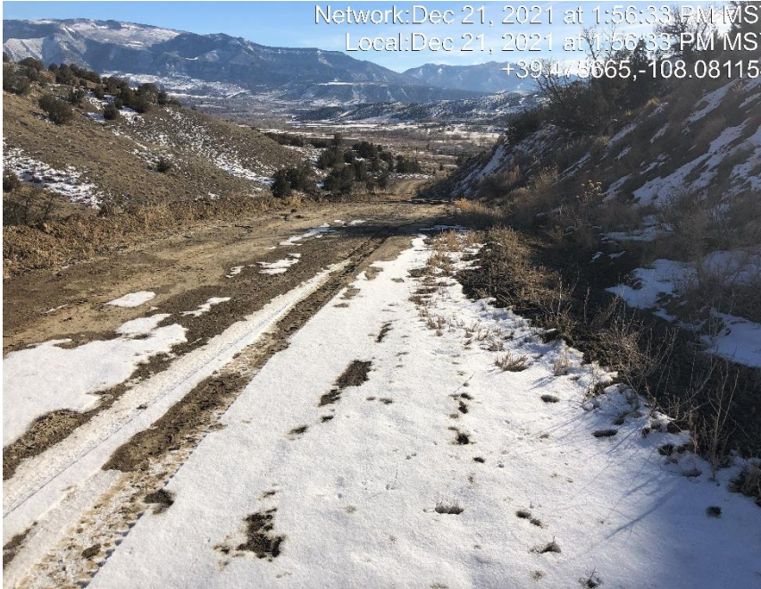
Photo #5479 Insufficient tracking BMP located at entrance to location.
