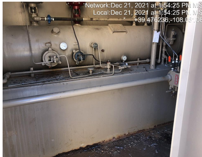
Photo #5476 Storage tank is located under horizontal separator.
