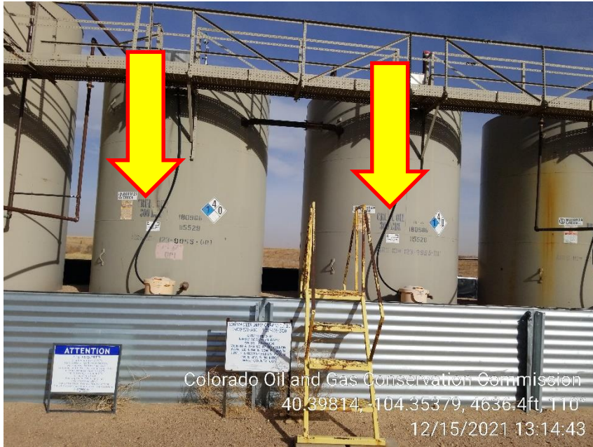
Photo 5 – Tank Battery – Content and Capacity Labels
