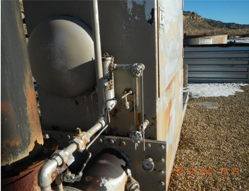
**The sight glass located on the side of the unit indicates the storage tank is full of an unknown fluid.**
