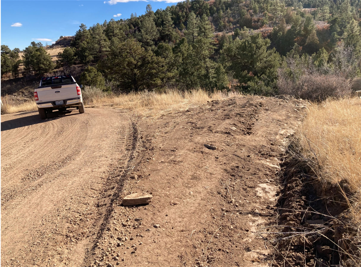
A WATER CALLOUT WAS INSTALLED TO REDUCE THE VOLUME OF RUN OFF ON THE ROADWAY SURFACE.
