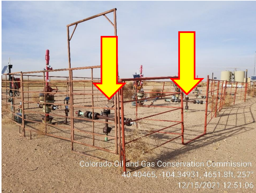
Photo 1 – Wellheads – Unmarked Risers
