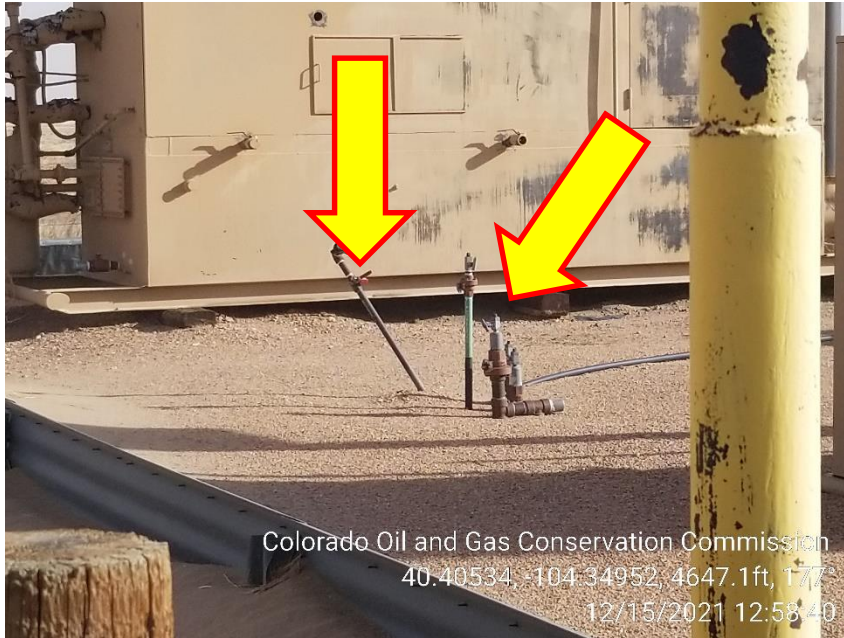
Photo 11 – Unmarked Risers at Separators
