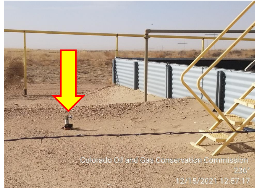
Photo 6 – Unmarked Riser
