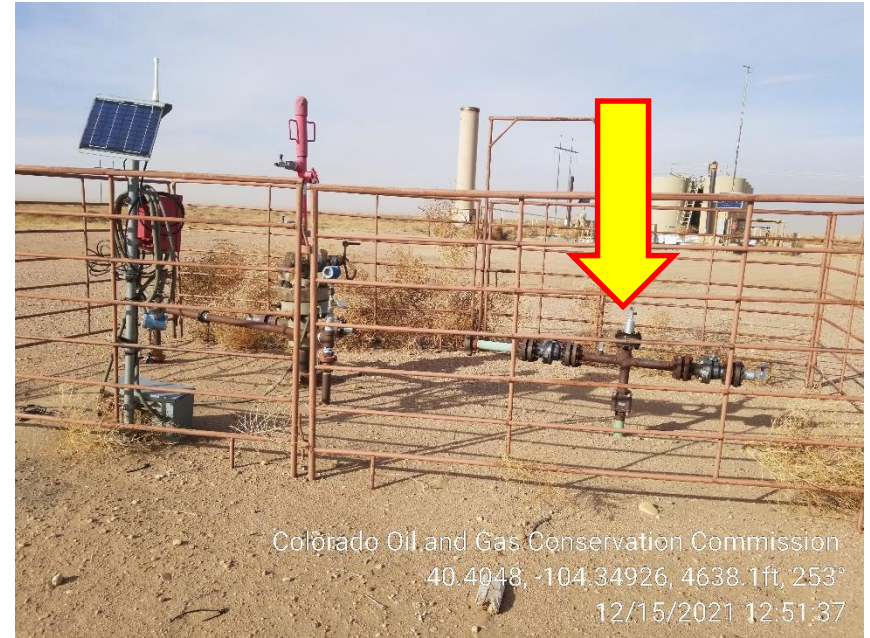
Photo 2 – Wellheads – Unmarked Risers
