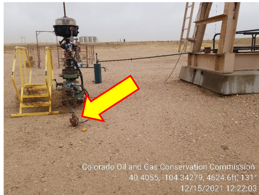
Photo 4 – Unmarked Riser at Pumping Unit Wellhead
