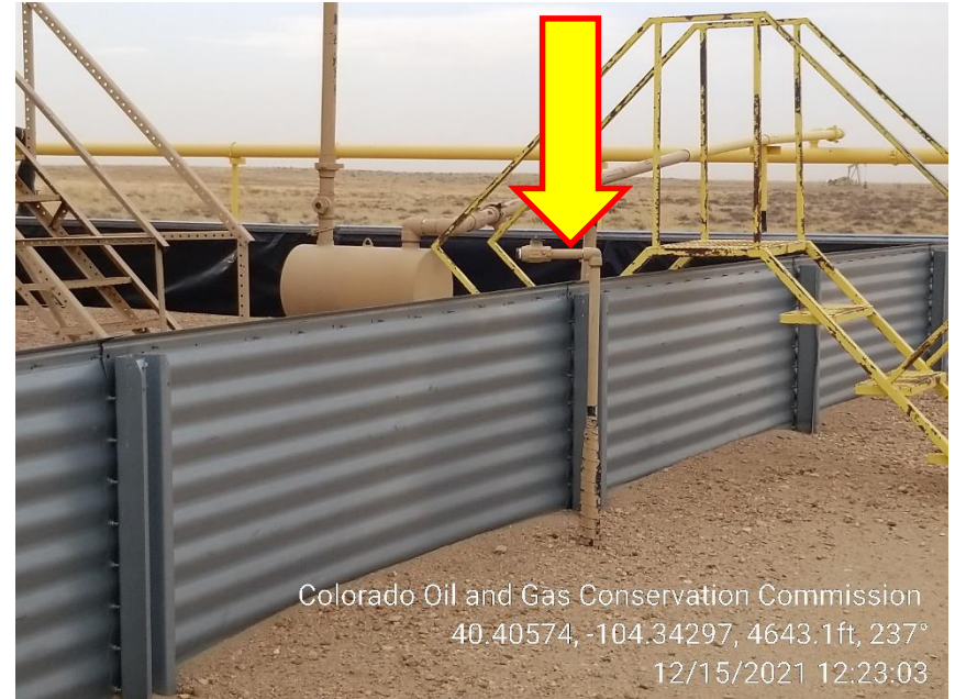
Photo 8 – Unmarked 1" Riser
