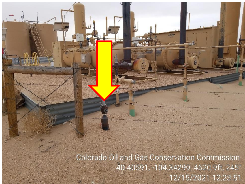
Photo 11 – Unmarked Riser
