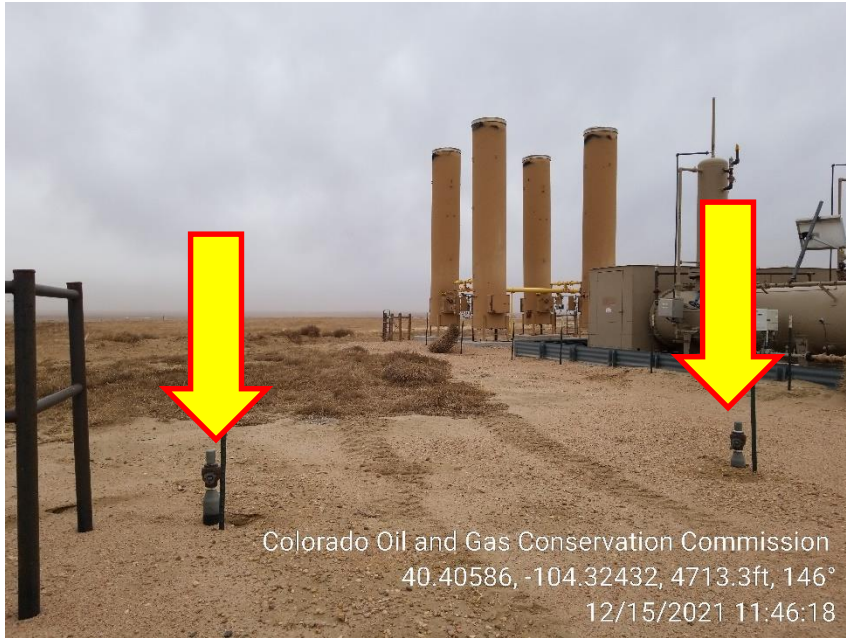
Photo 7 – Unmarked Risers
