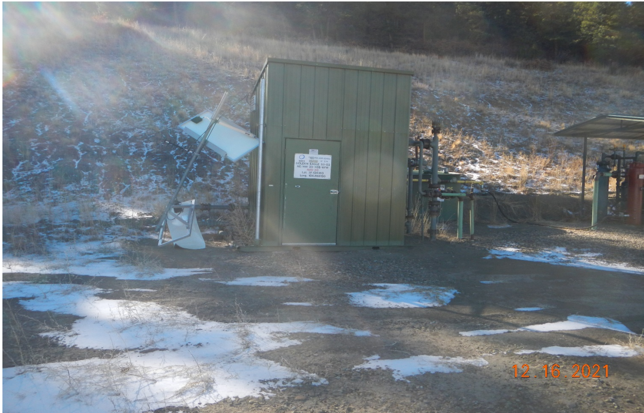
Photo 4. The solar panels at the meter shed have blown over.
