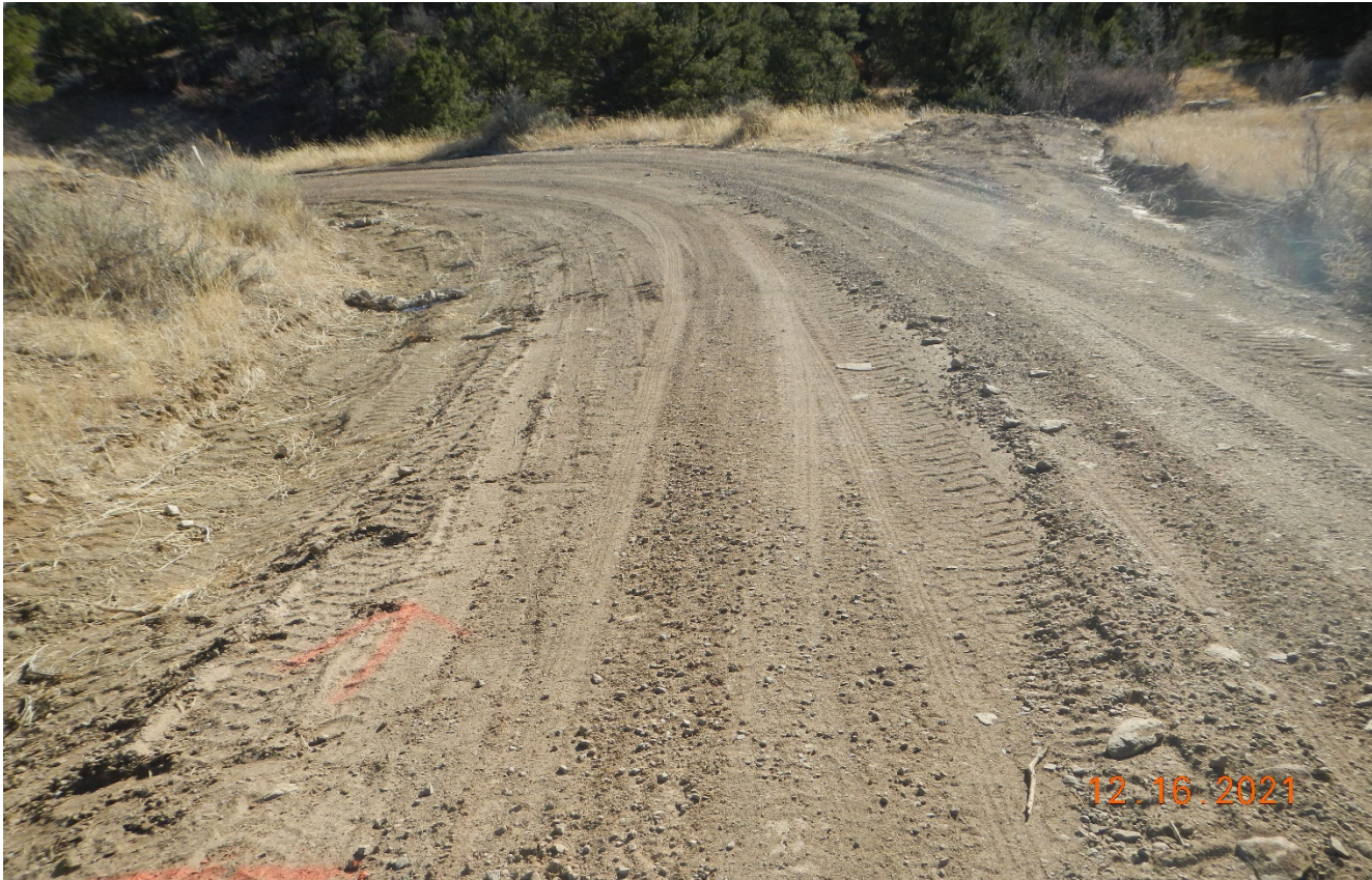
Photo 1. The erosion along the road side has been repaired.
