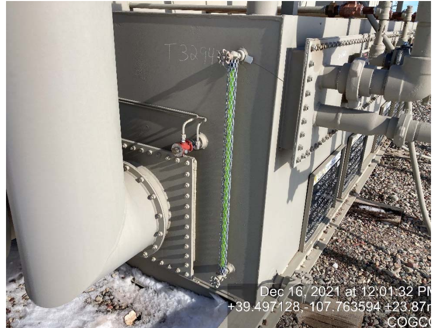
Storage tank lacking labeling/sight glass shows fluid
