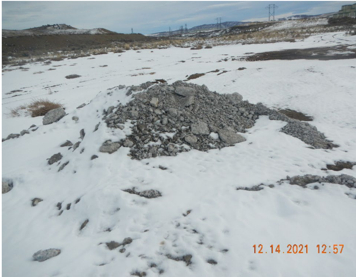
Photo #12 pile of cement. This pile can not be incorporated in any backfill
