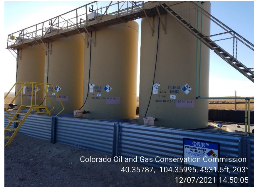
Photo 10 – West Side Tank Battery
