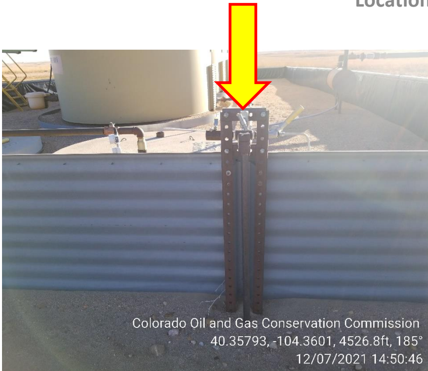
Photo 11 – West Side Tank Battery – Unmarked Risers
