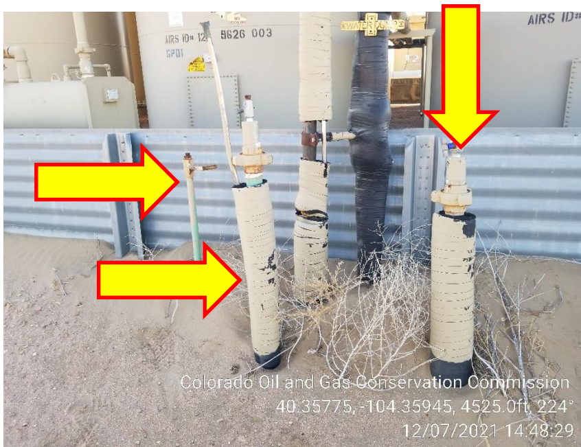
Photo 9 – 41-44-31HZ Tank Battery (East Side) – Unmarked Risers
