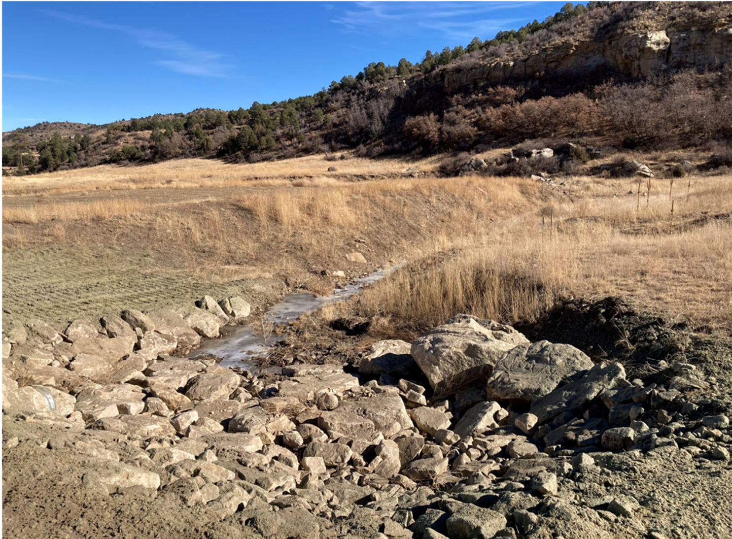
ARMOR WAS INSTALLED IN THE DITCH LINE THAT RECEIVES STORMWATER FROM THE LEASE ROAD AND IN FRONT OF THE CULVERT OUTLET FOR PERMANENT STABILIZATION AND EROSION CONTROL.
