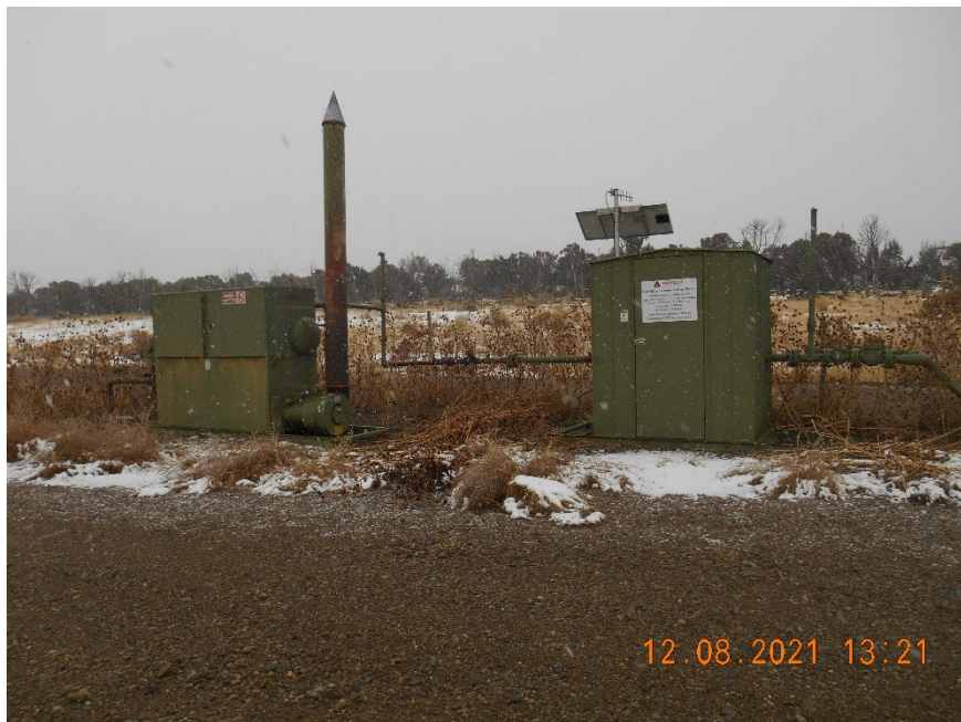
Separator and meter housing
