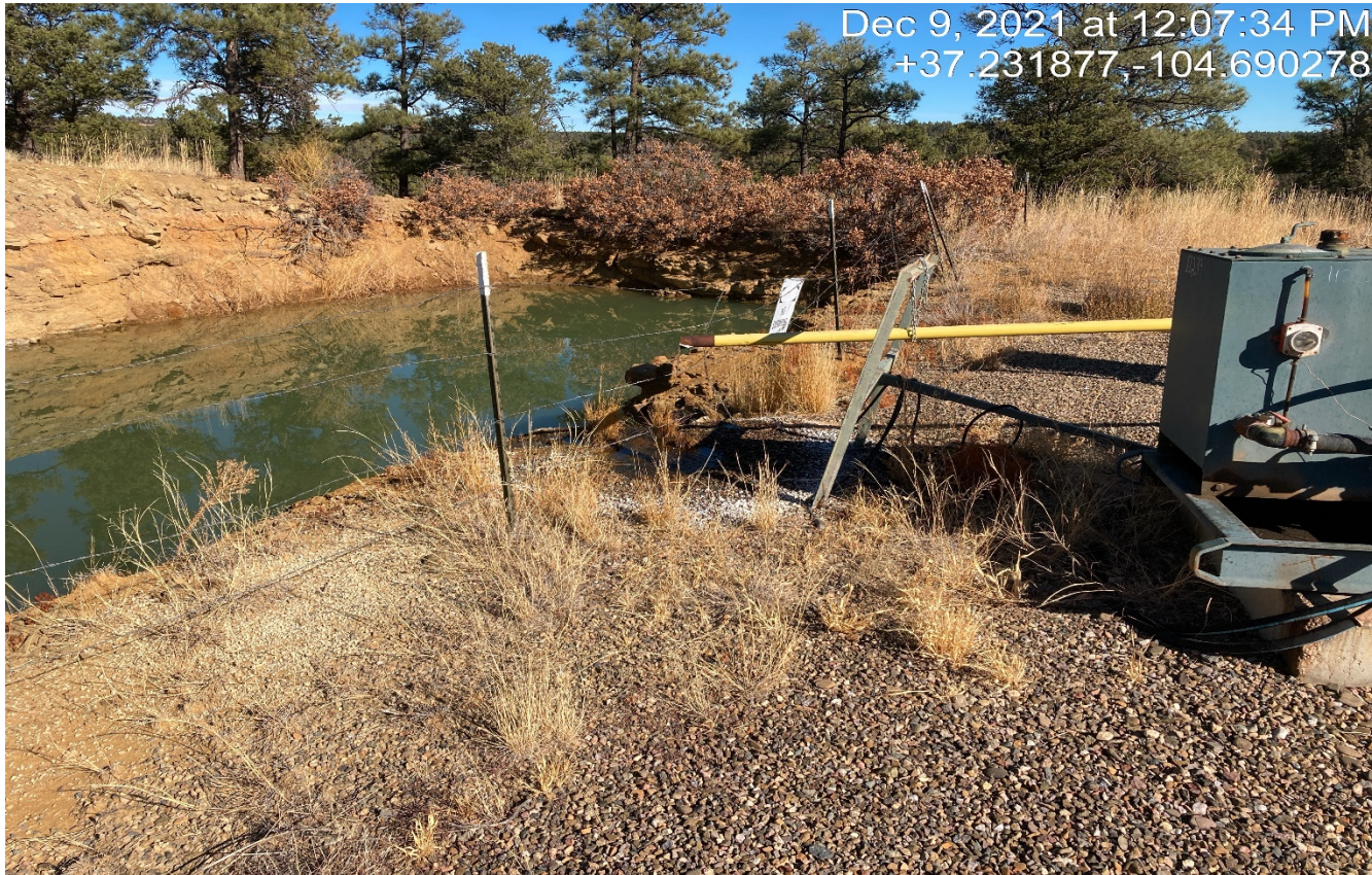
Photo 3. The PW pipe is not long enough to reach the pit. Previous corrective action was not performed.
