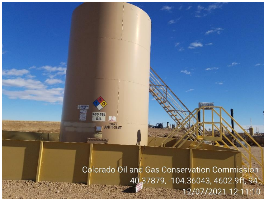
Photo 3 – Tank Battery
