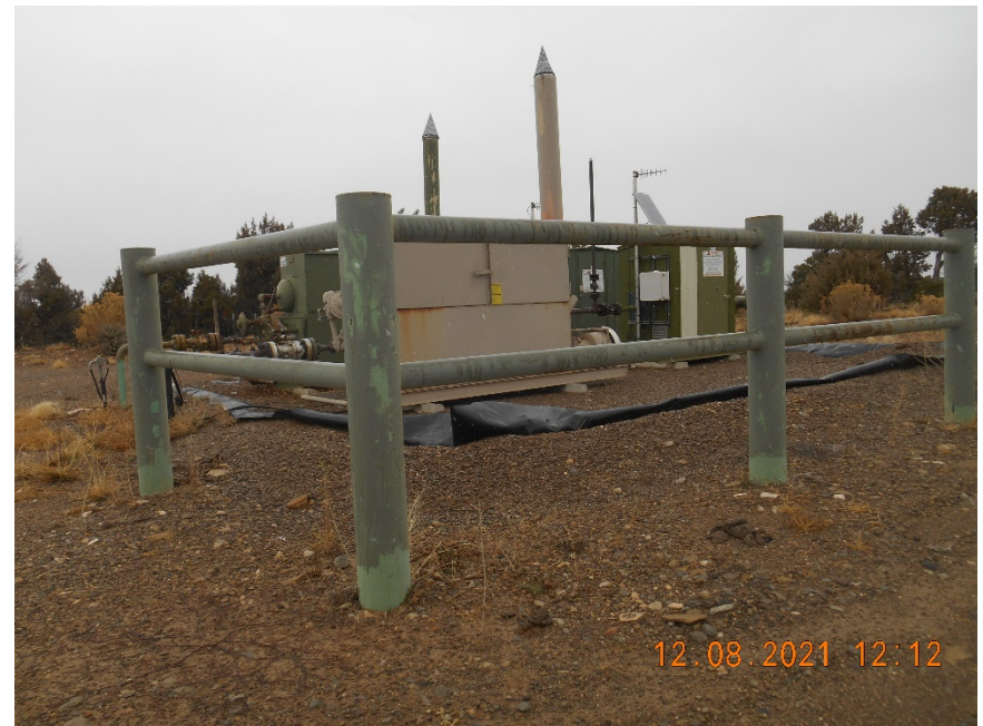
Separators and Meters with sign
