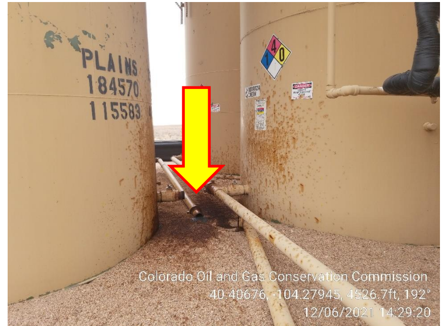
Photo 2 – Stained Soil at Tank Loadline
