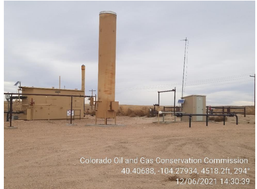
Photo 6 – Separator, ECD, and Gas Meter
