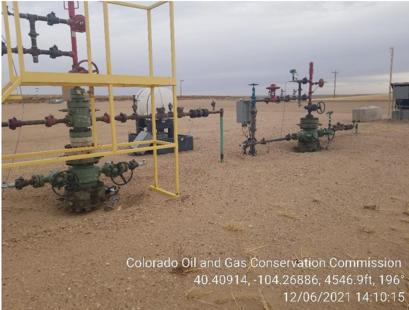
Photo 3 – 34-12 and 44-41 Wellheads – Missing Wellhead Signs
