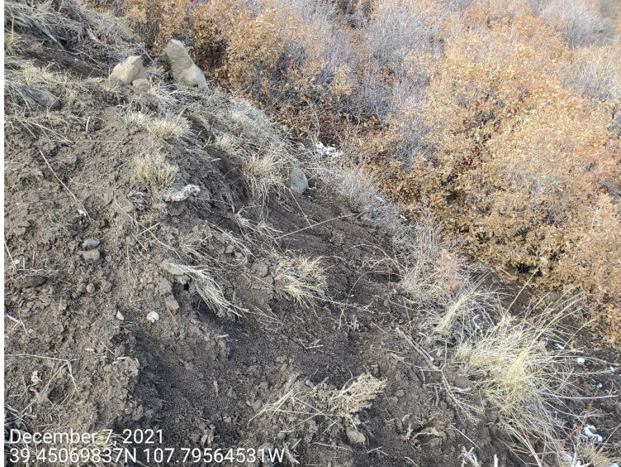
Photo 10: Photos examples showing control measures to protect and stabilize the topsoil stockpiles on the Location remain missing or insufficient.
