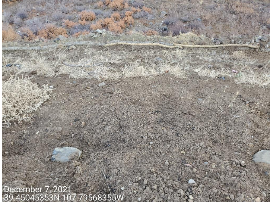
Photo 6: Photos examples showing control measures to protect and stabilize the fill slopes of the Location remain missing or insufficient; degradation has persisted.
