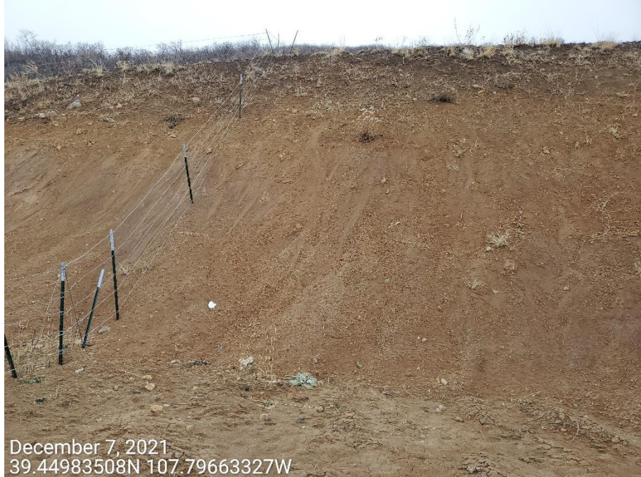
Photo 8: Photos examples showing control measures to protect and stabilize the cut slopes of the Location remain missing or insufficient; degradation has persisted.
