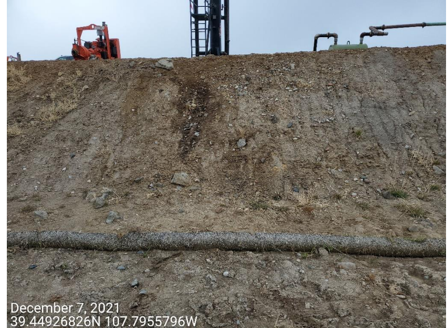
Photo 2: Photos taken from the southeast end of the Location, facing north. Photos show grey discolored/impacted soils observed on the fill slopes, and flat areas where the pit previously existed. Unclear what the observed materials are.
