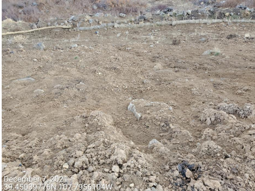
Photo 7: Photos examples showing control measures to protect and stabilize the fill slopes of the Location remain missing or insufficient; degradation has persisted.
