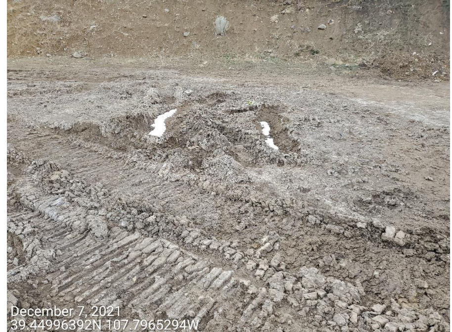
Photo 16: Photos show control measures to stabilize the production areas, and mitigate tracking and sediment transport are missing or insufficient.
