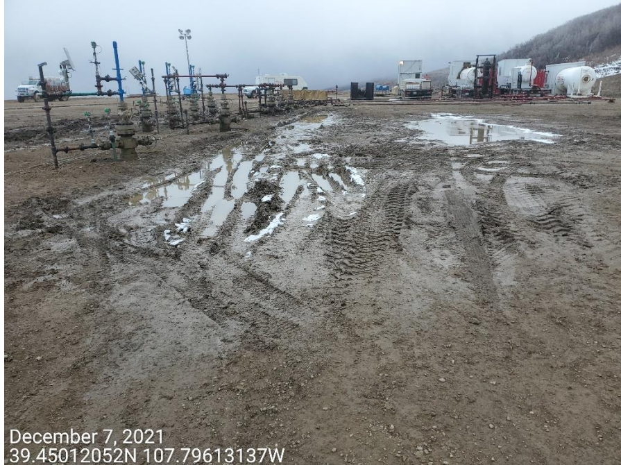
Photo 15: Photos show control measures to stabilize the production areas, and mitigate tracking and sediment transport are missing or insufficient.
