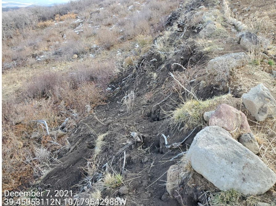
Photo 11: Photos examples showing control measures to protect and stabilize the topsoil stockpiles on the Location remain missing or insufficient.
