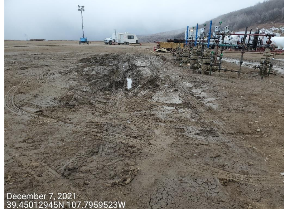
Photo 15: Photos show control measures to stabilize the production areas, and mitigate tracking and sediment transport are missing or insufficient.
