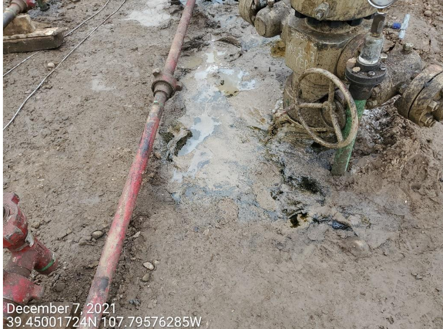
Photo 4: Photos examples showing impacted/stained materials observed around the wells.
