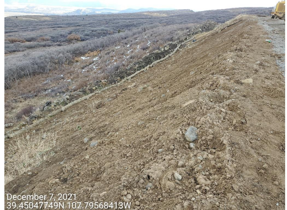
Photo 6: Photos examples showing control measures to protect and stabilize the fill slopes of the Location remain missing or insufficient; degradation has persisted.
