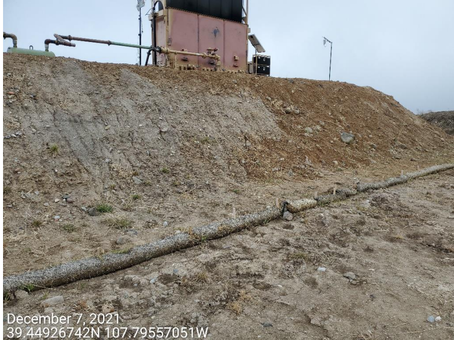
Photo 3: Photos taken from the southeast end of the Location. Photos show grey discolored/impacted soils observed on the fill slopes, and flat areas where the pit previously existed. Photo right shows a pile of grey material (possibly drilling mud) observed on the perimeter of the pad above the slopes in photo 2. Unclear what the observed materials are.
