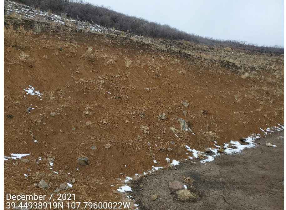
Photo 8: Photos examples showing control measures to protect and stabilize the cut slopes of the Location remain missing or insufficient; degradation has persisted.
