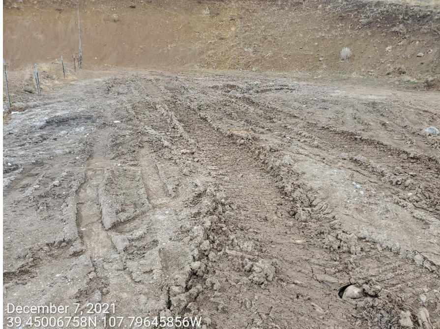
Photo 16: Photos show control measures to stabilize the production areas, and mitigate tracking and sediment transport are missing or insufficient.
