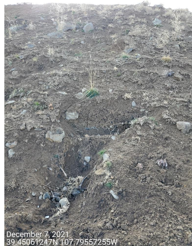
Photo 7: Photos examples showing control measures to protect and stabilize the fill slopes of the Location remain missing or insufficient; degradation has persisted.
