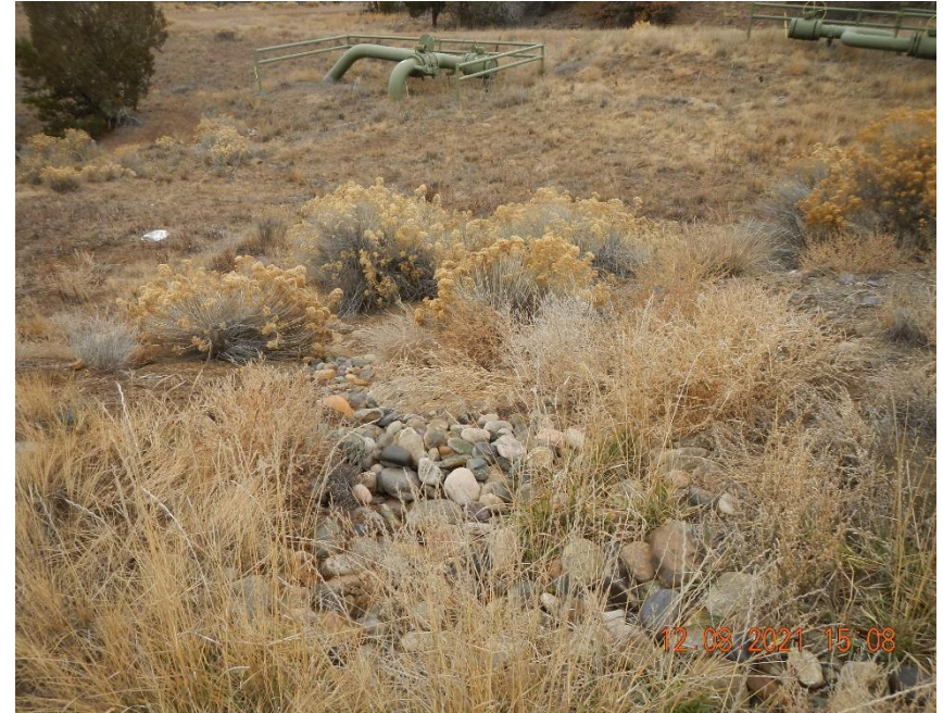
Rip rap run down along western edge of the location.
