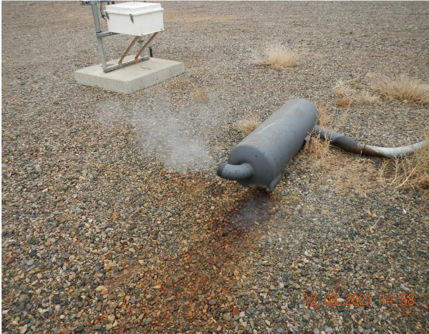
Stained gravel near prime mover exhaust.
