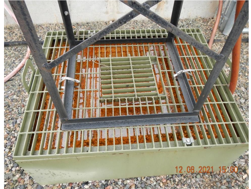
Secondary containment for lube oil container is almost full.
