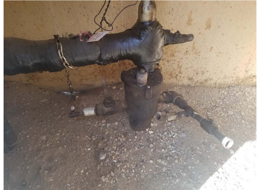
Photo 2. No bradenhead access apparent.
