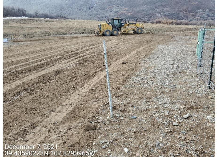
**Photo 2:** Photos taken from the east end of the Location. Photos show that though work to address the compliance issues is in process at time of inspection, control measures to stabilize the production areas and to mitigate tracking and offsite sediment transport remain missing or insufficient. Operator on site observed re-grading tracking/ruts on the production areas; re-grading alone insufficient to address stabilization, tracking and offsite sediment transport.
