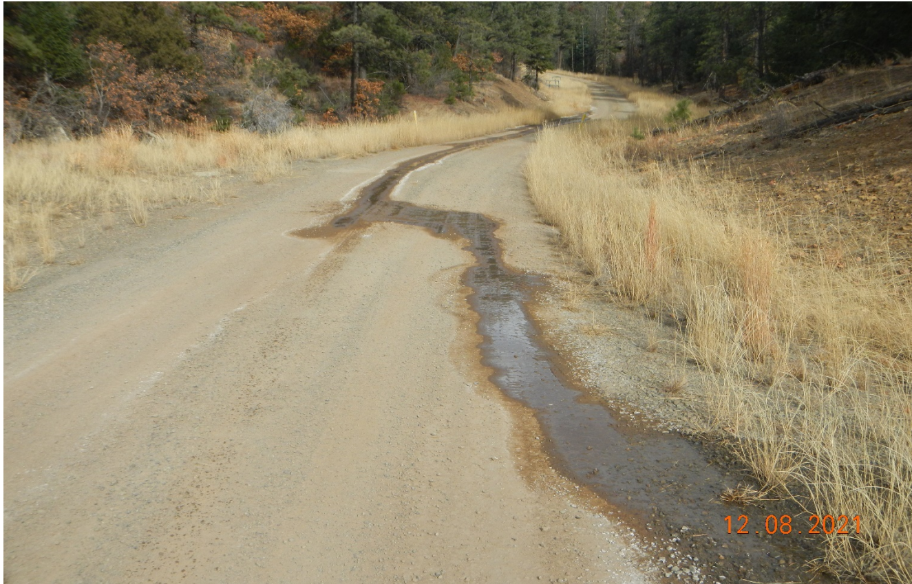
Photo 2. Standing at the well site facing north toward the road. The source of the water flowing down the road is unknown and should be inspected by the operator.
