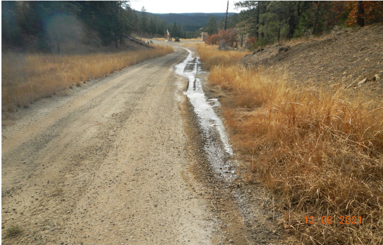
Photo 1. Facing southwest along the access road. There is water draining down the road which needs to be properly diverted.
