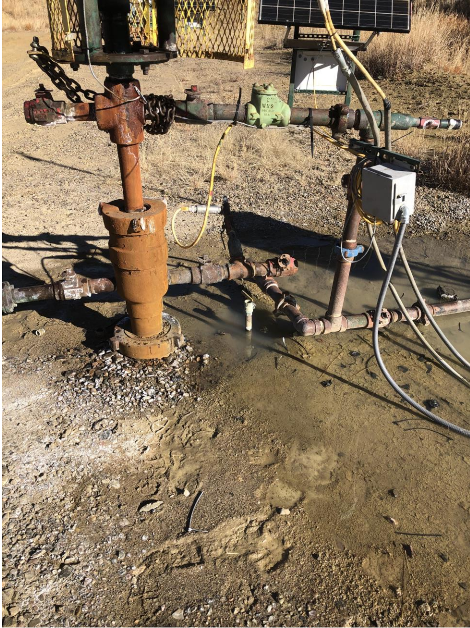
Provided access to bradenhead , to comply with new rule 341
