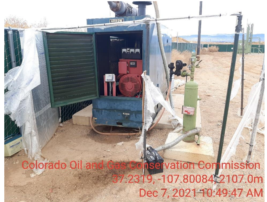
Photo 4 Stained soil from exhaust and motor
