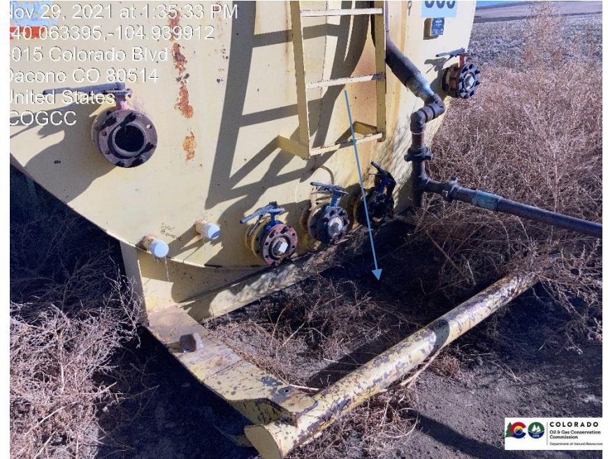
Pic 4 stained soil by tank that is on location.
