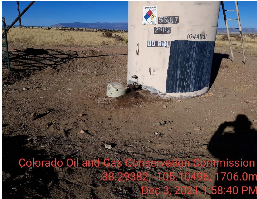
Photo 3 stained soil around crude oil load out line .
