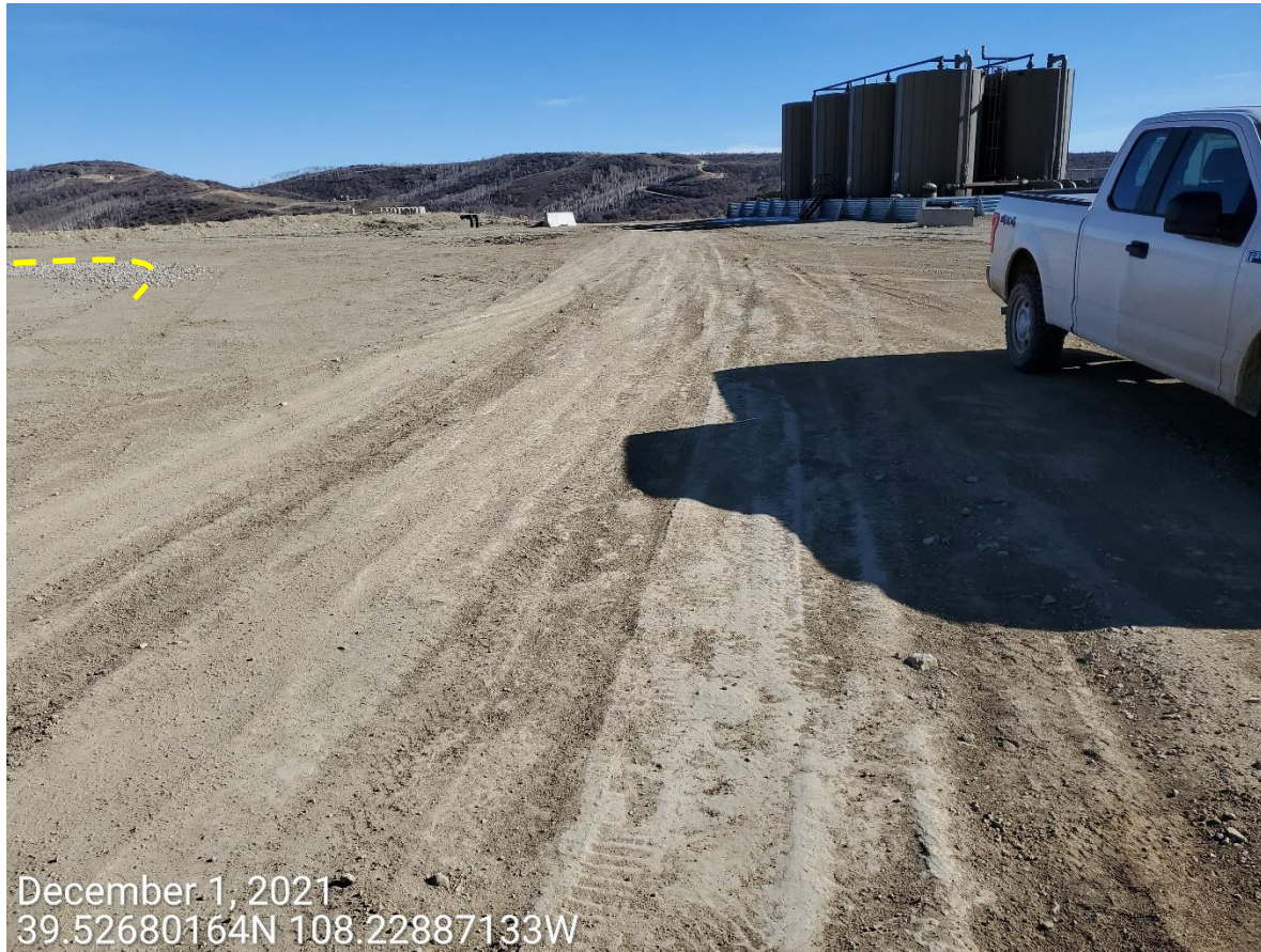
Photo 2: Photos taken from the Location, east. Photos show Operator placed gravel on select sections of the Location; from the western entrance leading around the well. Control measures to stabilize the entire Location, minimize tracking and offsite sediment transport per good engineering practices remain missing or insufficient.
