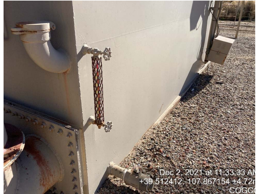
Glycol vessels lacking labeling
