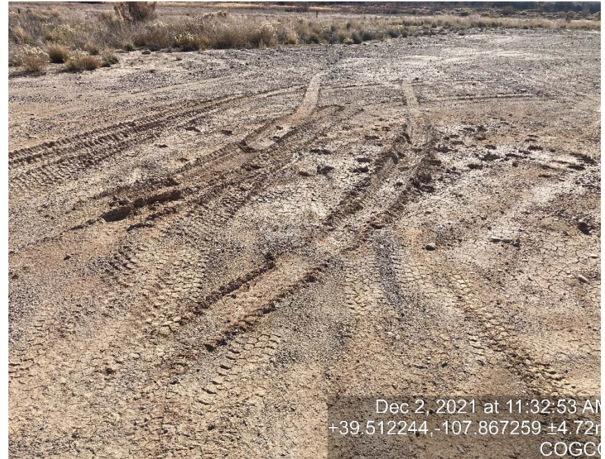
Lack of stabilization/compaction
