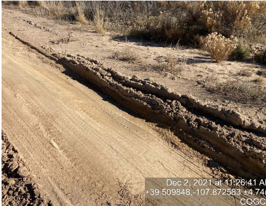
Access road lack of stabilization/compaction
