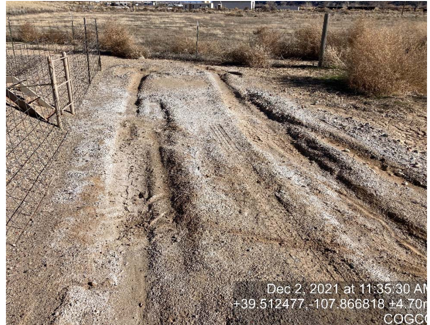
Lack of stabilization/compaction
