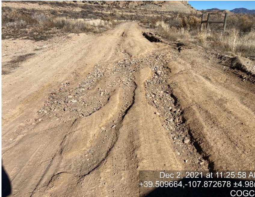
Access road lack of stabilization/compaction
