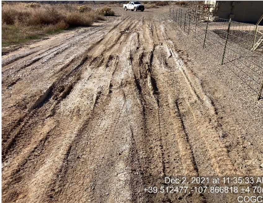
Lack of stabilization/compaction
