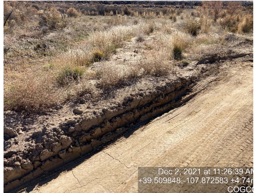
Access road lack of stabilization/compaction
