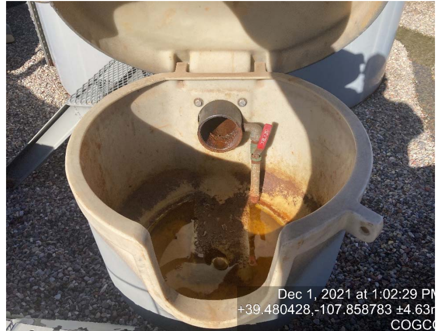
Load lines missing bull plugs/caps
