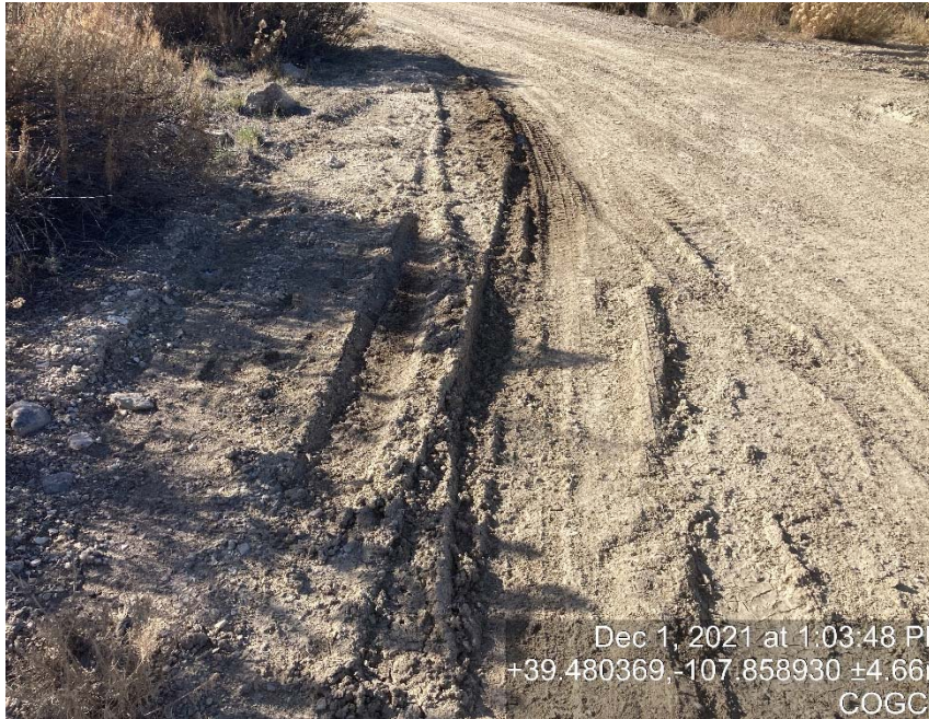
Location lack of stabilization/compaction
