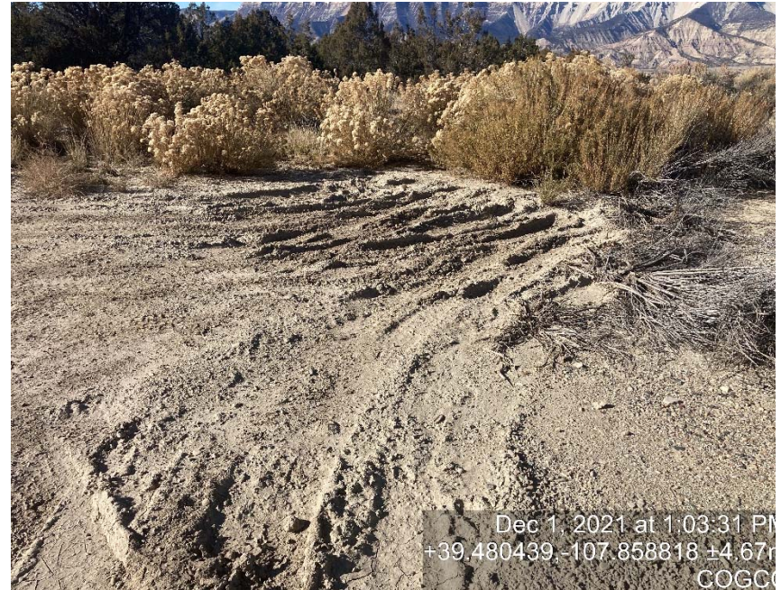
Location lack of stabilization/compaction
