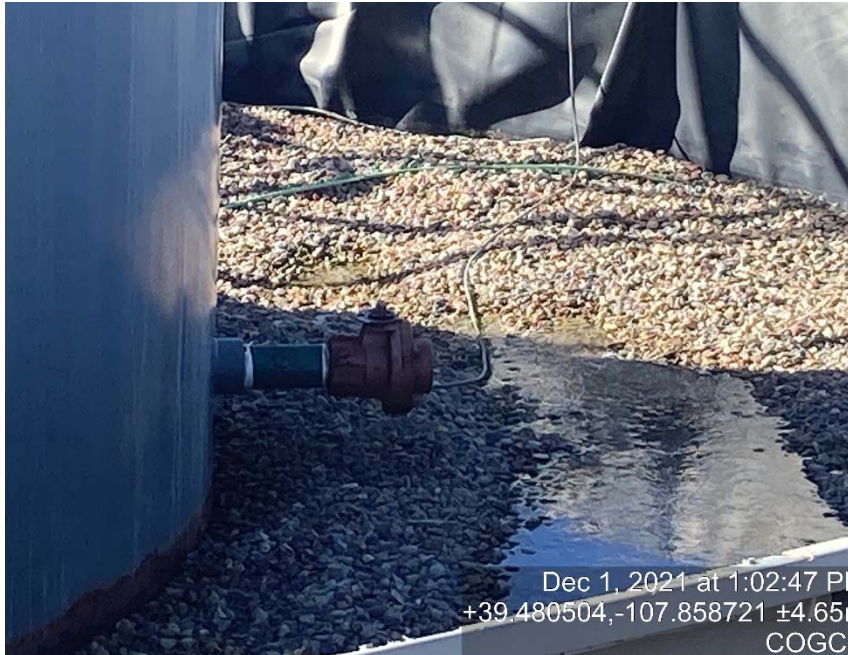
Load lines missing bull plugs/caps
