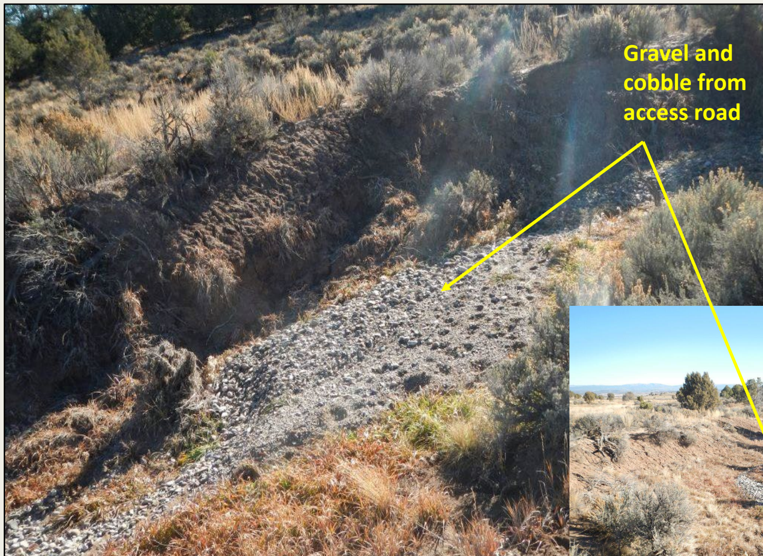
Photo 8. View of area approx. 50 ft down-slope of culvert outlet, where significant volumes (approx. 75ft long, 4-6 ft wide, and 4-6 inches deep) observed within the streambed.
