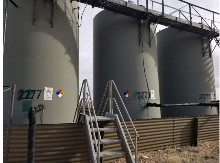
Photo 2. No capacity on tank labels.
