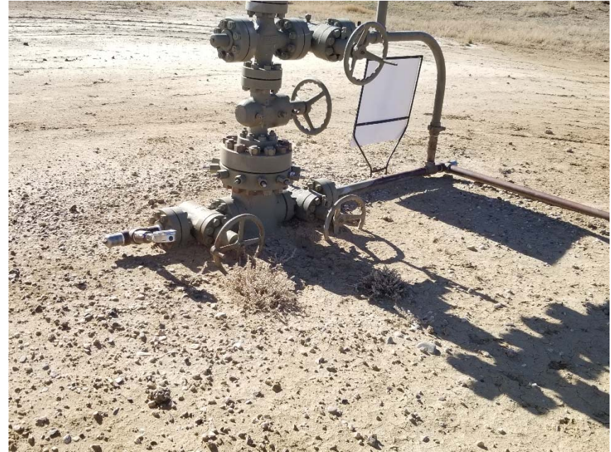
Photo 2. No bradenhead access apparent.
